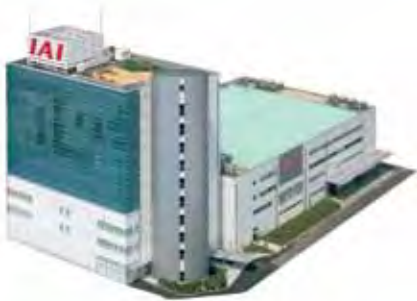
IAI Headquarters On the windows of the newly constructed headquarters spell out the character for 'heart' in Japanese. This character is rich and meaningful, symbolizing the heart, spirit, attention and sincerity of IAI's commitment to the users of IAI products.
