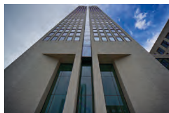
Opera Tower Frankfurt, Germany
