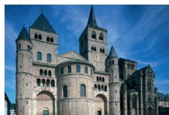
Liebfrauenkirche (Cultural Heritage) Trier, Germany
