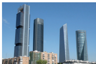
4 Towers Business Area Madrid, Spain
