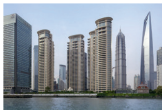
Tomson Riviera Apartment Towers Shanghai, China
